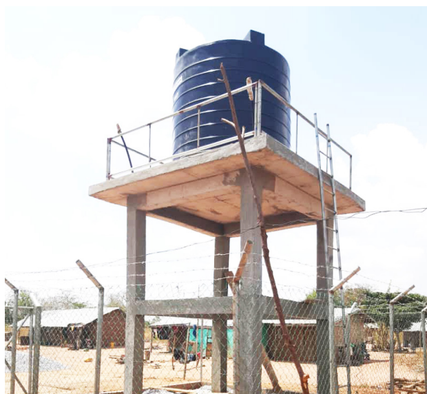
Storage tanks are provided to ensure access to water during dry periods
